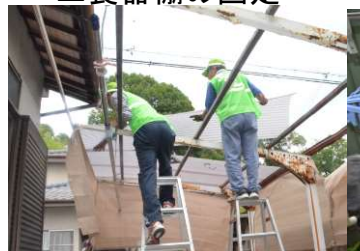
▲波板の張替え
