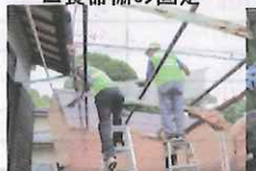
▲波板の張替え
